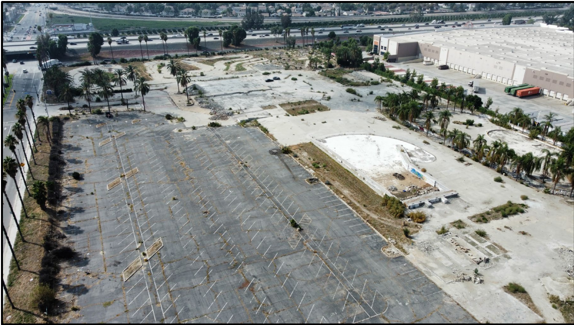
Plate 3.2–1: Drone overview of the subject property, facing south.
