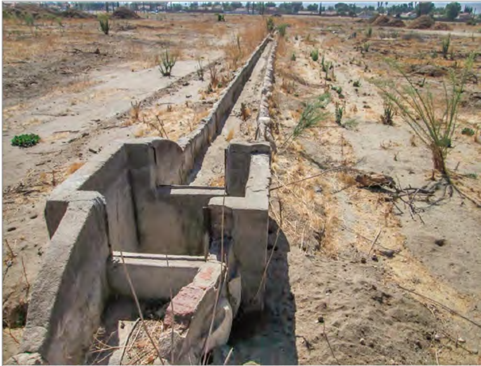
View south of flume showing brick-and-mortar weir (flow control structure)
