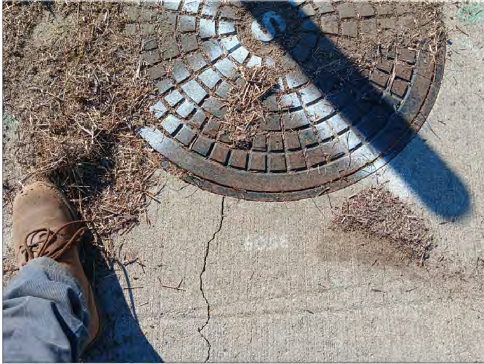
Photograph 5: Underground wastewater underground line, plan view.
