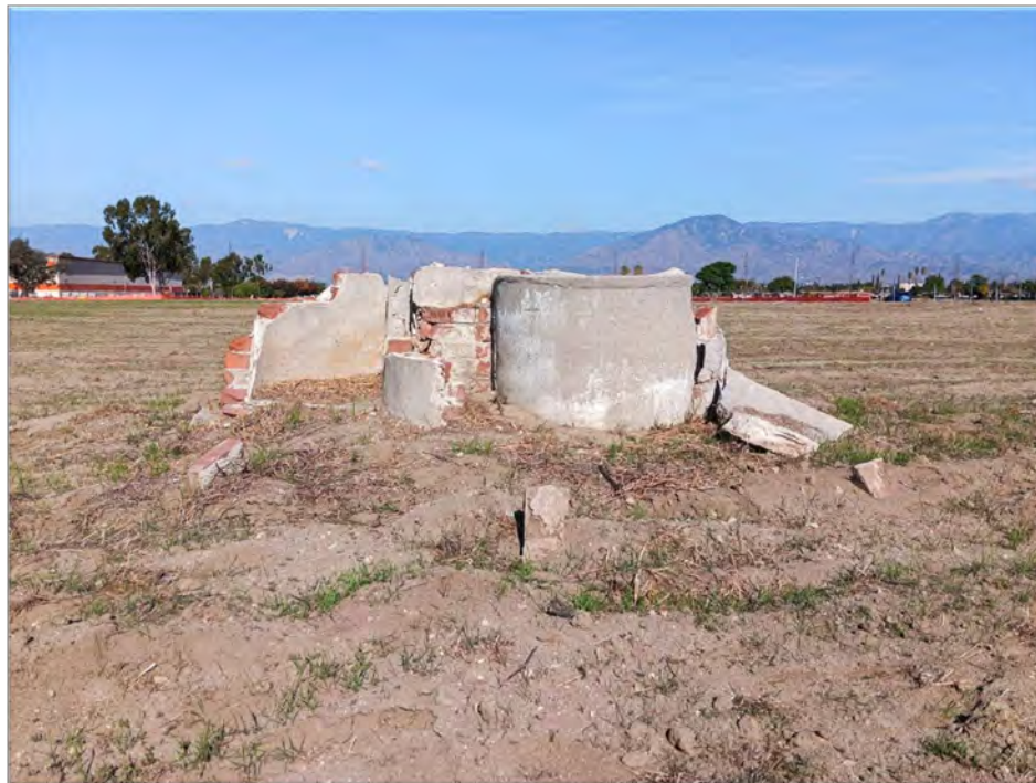
Photograph 8: Feature A, view to the north.
