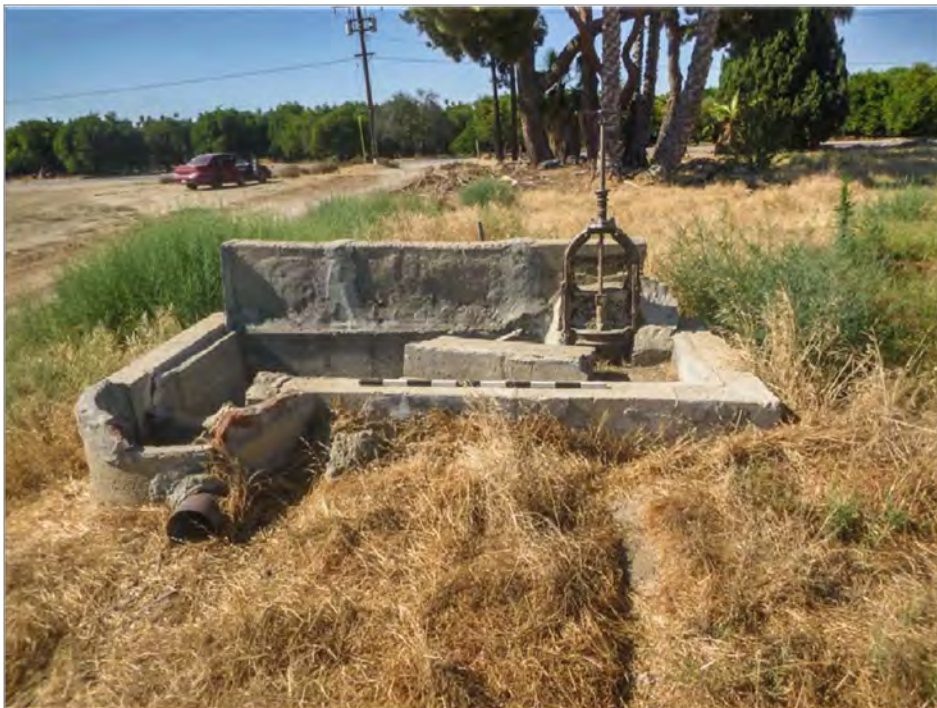
Figure 5-4 Overview of weir (Æ-3895-2H) view looking south.
