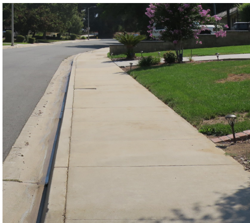
Match new concrete to adjacent concrete.
