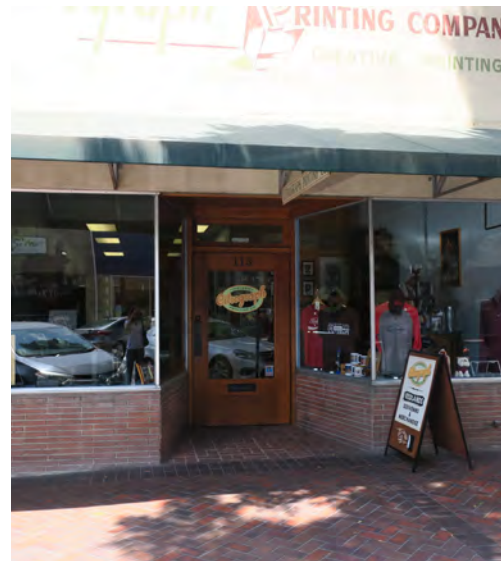
An example of a recessed storefront entrance, a common characteristic of the city’s downtown commercial buildings.
