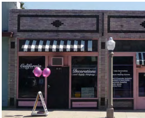
An example of a one-story commercial building, typical of Redlands' downtown commercial development.
