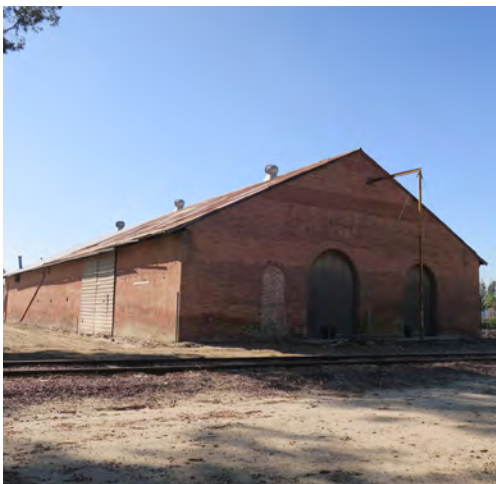
Brick is a prominent material in Redlands' industrial architecture.
