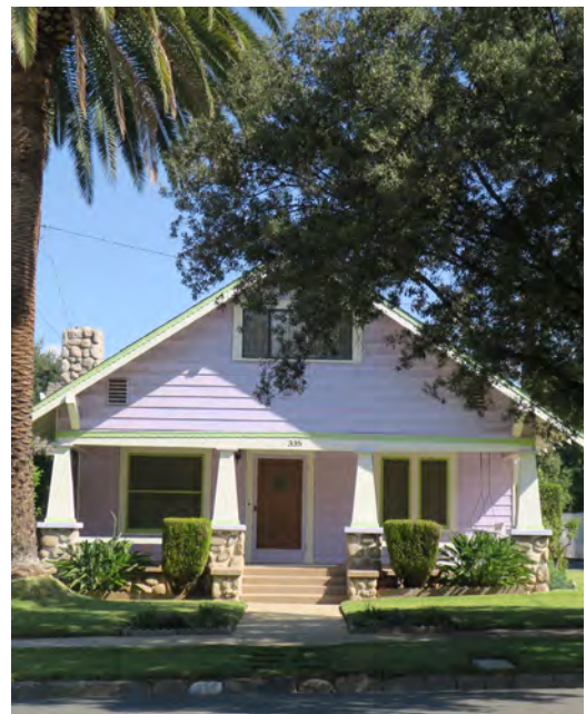
An full-width entrance porch is a prominent feature of houses in Redlands’ in pre-war neighborhoods.
