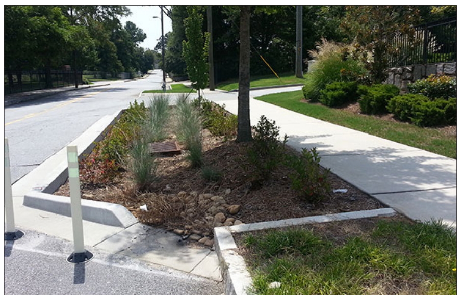
A break in the curb allows water to flow into planters.
