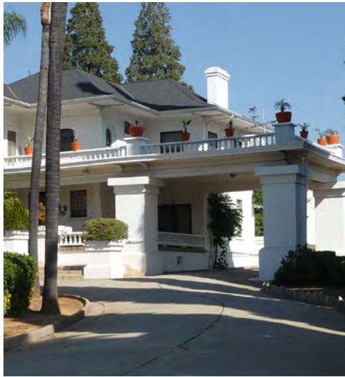
This porte-cochère is a historic ancillary structure that should be preserved.
