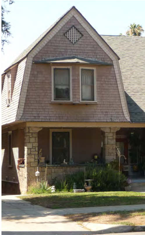
A gambrel roof is an important architectural feature of this Shingle style building and should be preserved.
