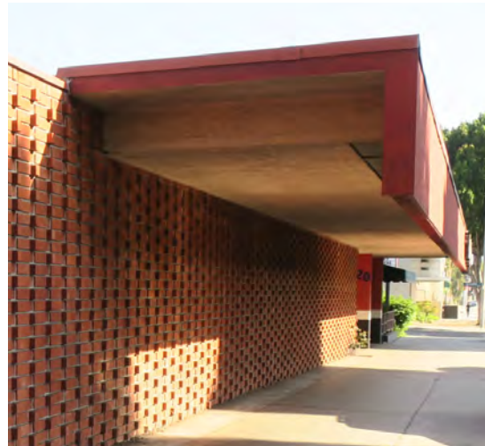
Routine maintenance will help prolong the life of this historic canopy.
