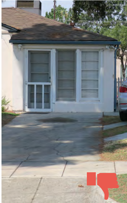
Avoid altering an ancillary structure in a way that obscures its historic character.
