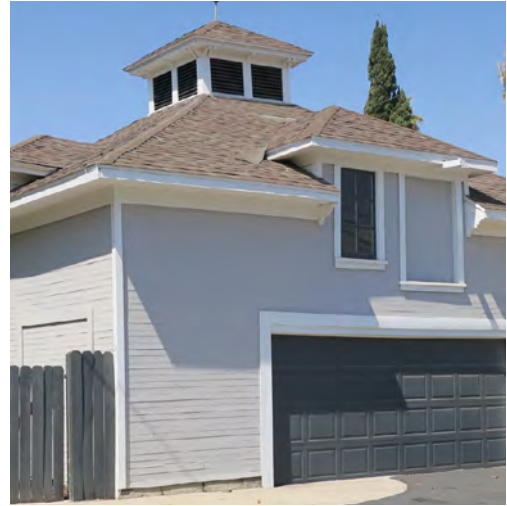
Restore a historic ancillary structure's missing components, such as historic garage doors or infilled openings.
