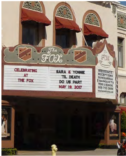
A historic sign, such as this theater marquee, is an important architectural feature that should be preserved.
