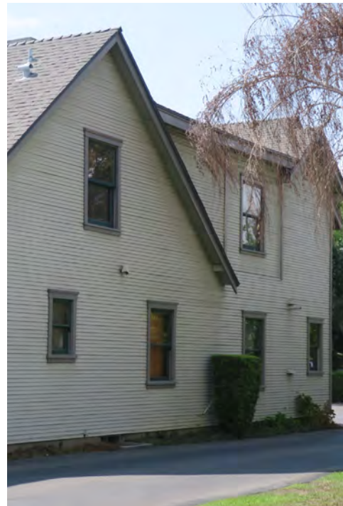
A historic rear addition.
