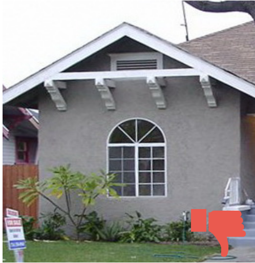
Avoid altering the size or shape of historic window openings on the primary façade of the building.
