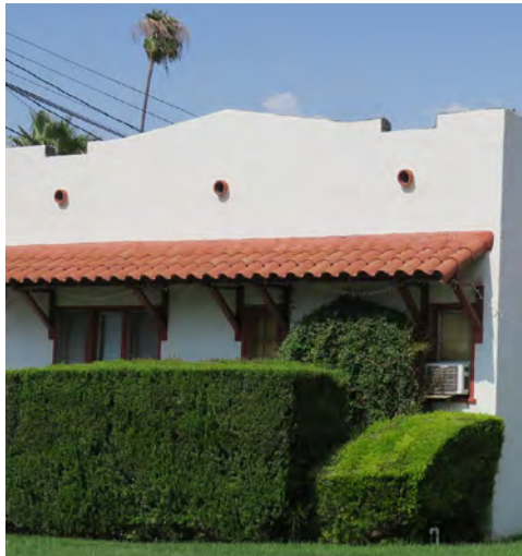
The clay tile awning on this house is an important historic accessory feature that should be preserved.
