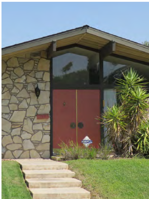
Paired wood slab doors are an important architectural feature of this Contemporary Ranch style house.
