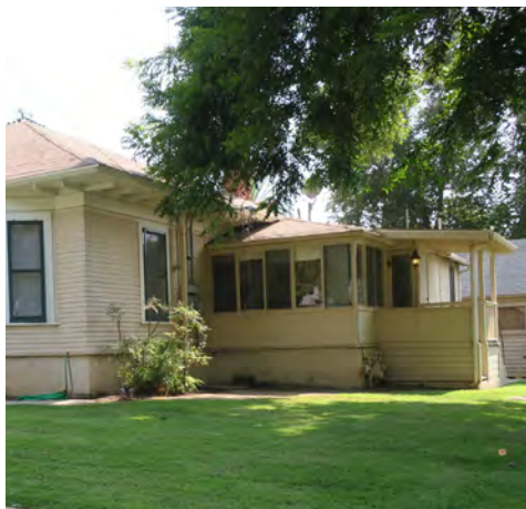
This porch addition tells the story of the building's development over time and should be preserved.
